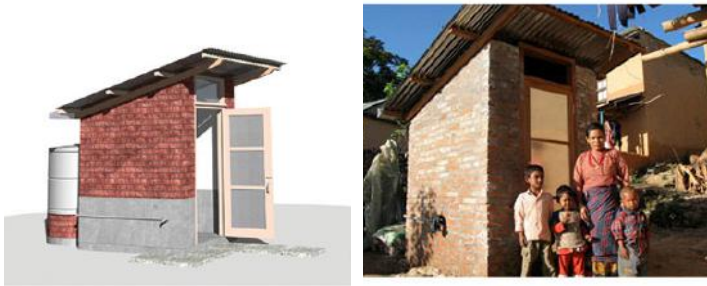
Figure 15. Design and in use sanitation facility. Source. Healthabitat (2016)
