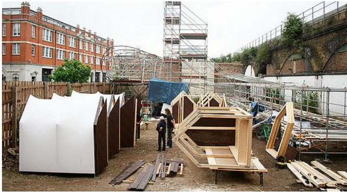
Figure 2. Lido during construction. Source. Southwarklido (2008)
